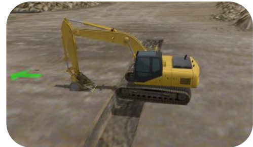
Trench Crossing using Boom Jacking
